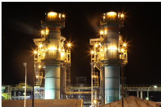
Sengkang Power Plant (Block 1) in South Sulawesi, Indonesia Initial CCGT 135 MW capacity
