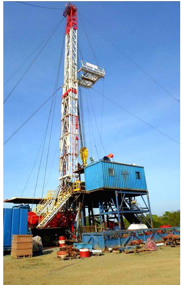
Drilling Rig for the Wasambo Drilling Program
