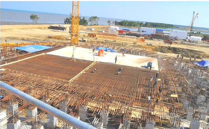
Sengkang LNG Site, South Sulawesi, Indonesia
