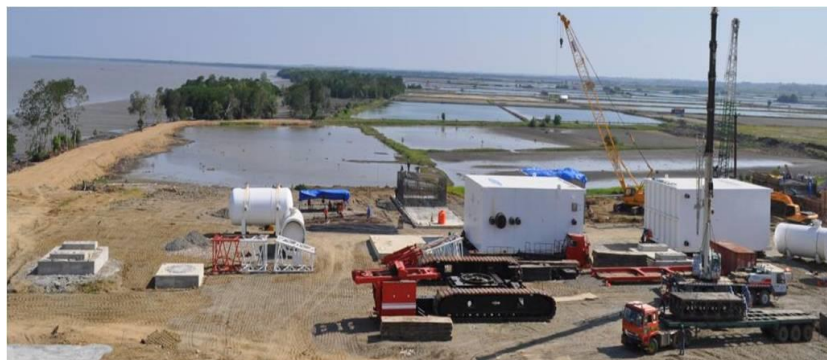
Main Processing Plant Area - Cold Boxes ready for placement
