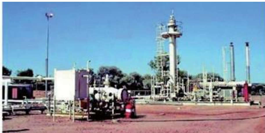
Gilmore Gas Plant, Australia
