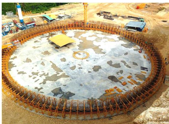
Slipform equipment assembling and rebar fixing in progress
